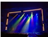
BLOOMINGTON, IL - The Bloomington Center for the Performing Arts (BCPA) in Illinois recently carried out a technical upgrade that has seen a number of GLP's impression Spot One and Volkslicht Zoom LED fixtures replacing traditional tungsten heads. Jason Reberski of JR Lighting Design supplied the fixtures. He recommended the Volkslichts as he uses them in his own production rental inventory.
